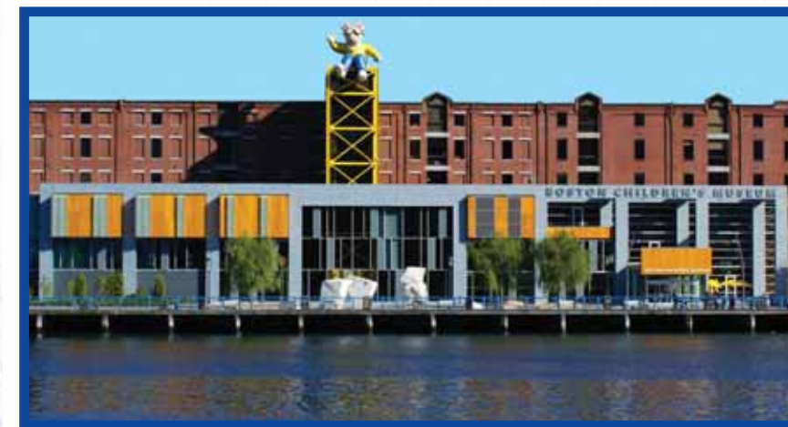
The museum's hangar style doors allow light and air into the building.
